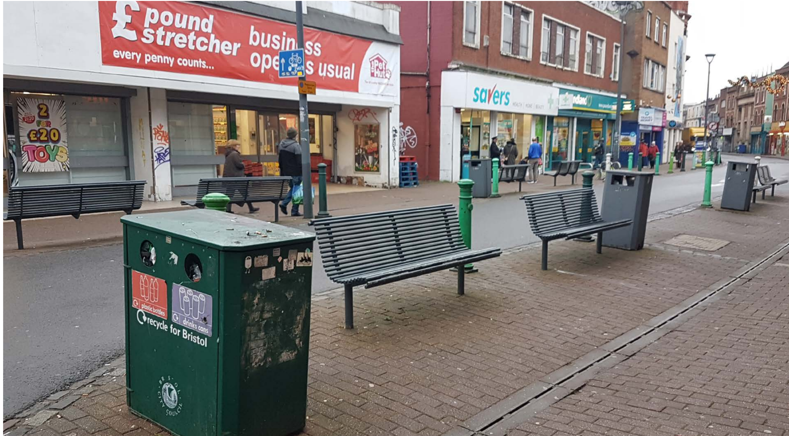
Cluttered street elements along the footpath
